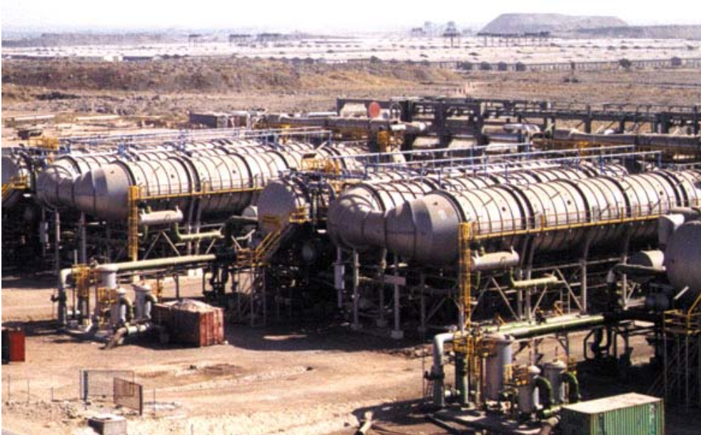
Fig. 5. Reliance refinery (India) – 4 \times \text{MED} 12,000 m 3 /d.
