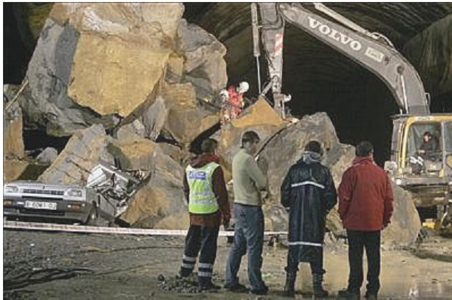
Fig. 2. Rockfall in late 2005 at a tunnel mouth in Northeast Spain resulting in one fatality [7].
