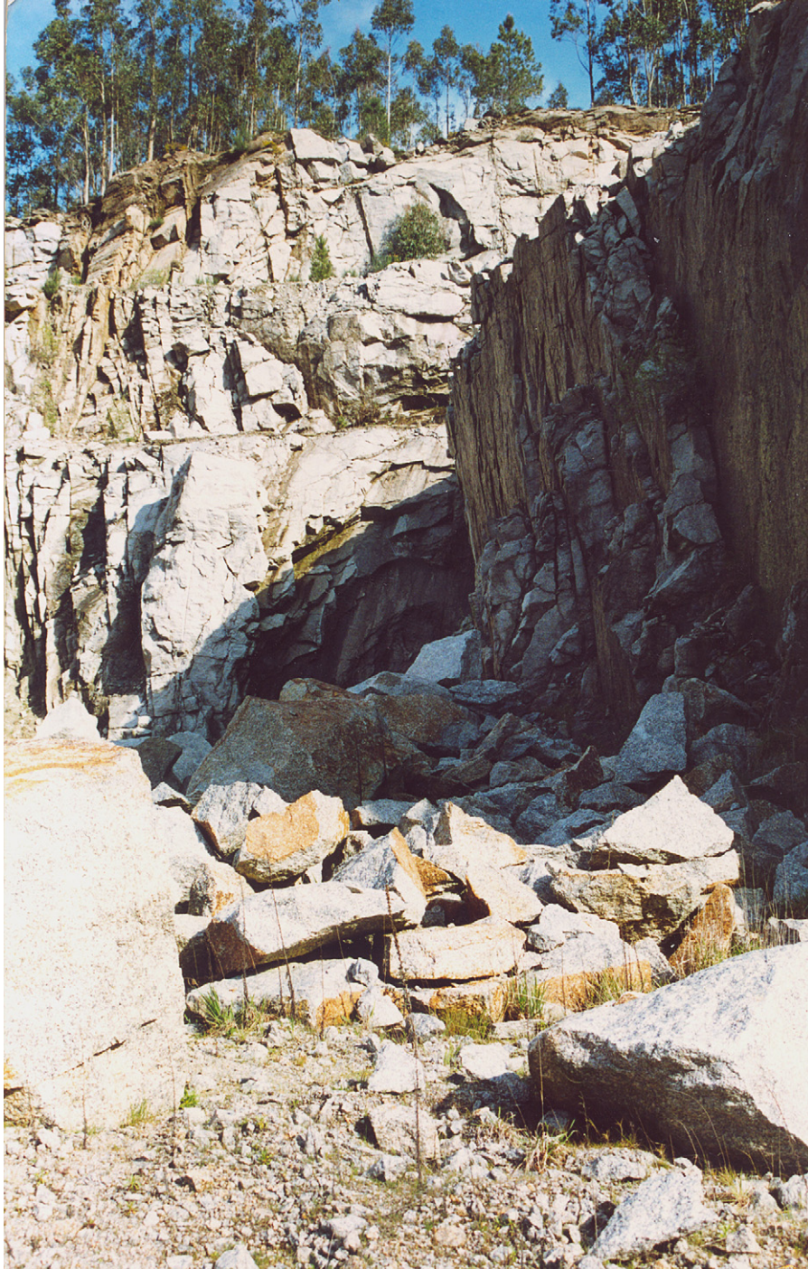
Fig. 20. Picture of a bench on Slope 2 of the aggregate quarry where toppling was recorded.
