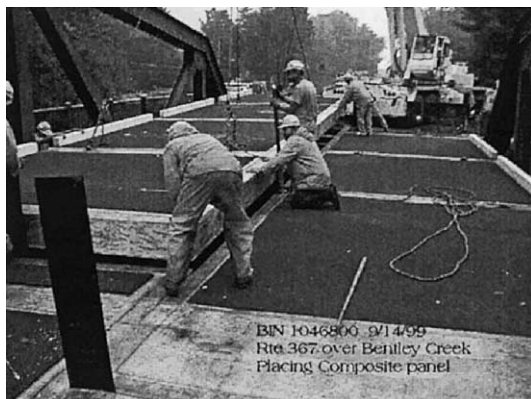
Fig. 2. Composite deck panels during installation.
